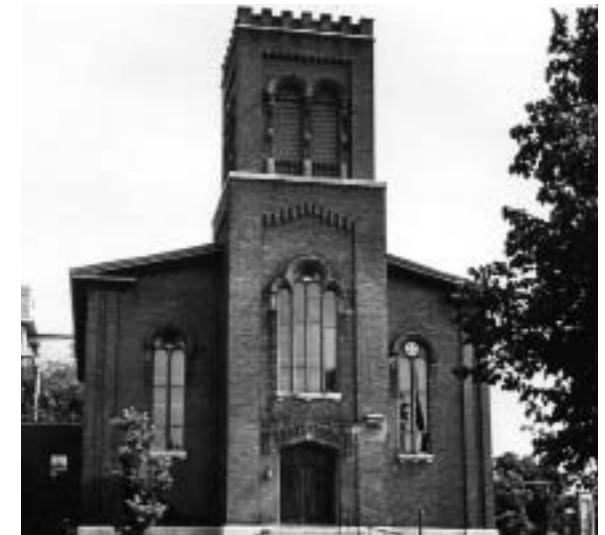
Old Brick, saved
